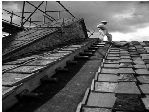
Retrofitting of the Basilica of San Francesco at Assisi, Italy
