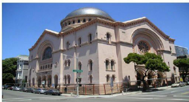
Exterior of the Sherith Israel Synagogue retrofitted with SMA devices
