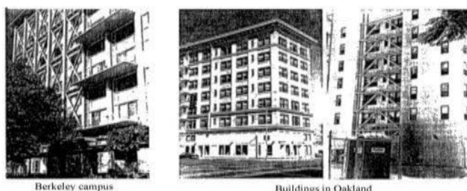
Use of sma bars to seismically upgrade buildings in Berkley and Oakland
